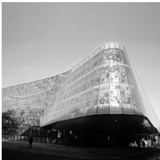
be provided with accurately engineered twisted roofs and flat roofs with twisted parts, where the glass panels were even insulated / laminated glass panels.
