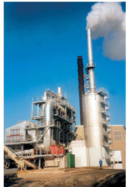
Wet Electrostatic Precipitator (WESP) behind a wood-chip dryer for the pellet production with a heat recovery system to feed into the district heating network, exhaust gas volume 78,000 Am 3 /h, temperature 110 °C, diameter 5,700 mm, recovered heat energy 4-4.5 MW/h, water outlet temperature 68 °C, heat recovery rate 35-45%
