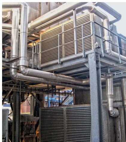
Water/Air-heat exchanger for pre-heating the combustion air of a dryer, air-volume 80,000 m 3 /h, heat output 1,400 kW/h
