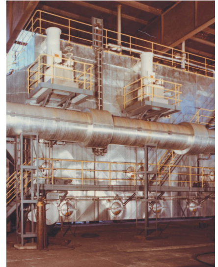
Dust collecting of cupola furnace waste gases
