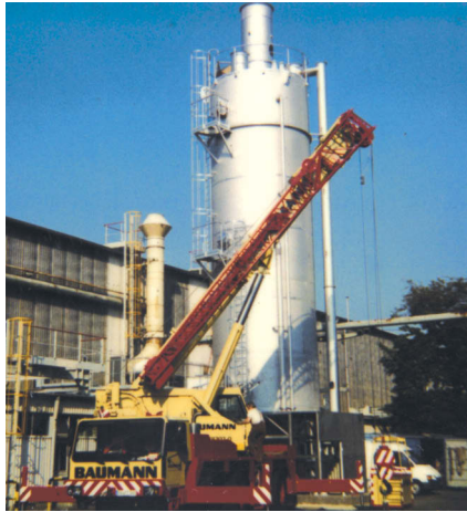
Vertical wet electrostatic precipitator for aerosol separation in the plastic industry
