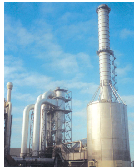
Waste gas cleaning system for 2 OSB-dryer System combination of quench, wet scrubber, dual wet electrostatic precipitator with stack up to 60 m
