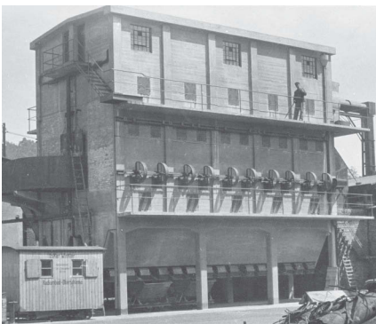
1924 Dry electrostatic precipitator for blast furnace gas
