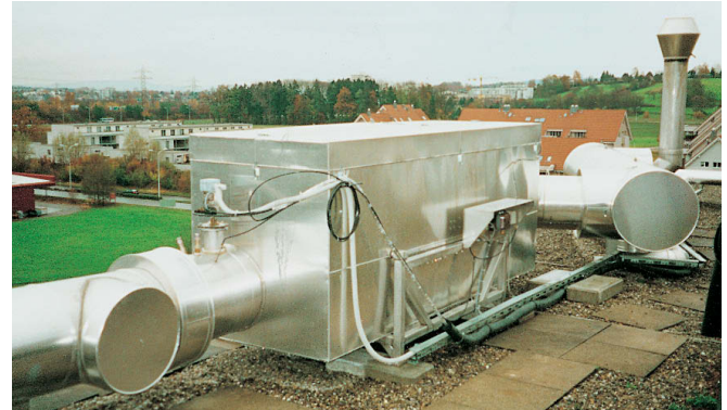
DeNO x unit for 2 diesel engines, 21,000 m 3 /h
