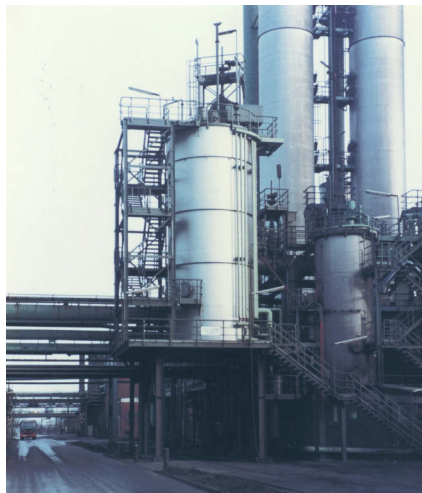
Vertical round type electrostatic precipitator for coke oven gas
