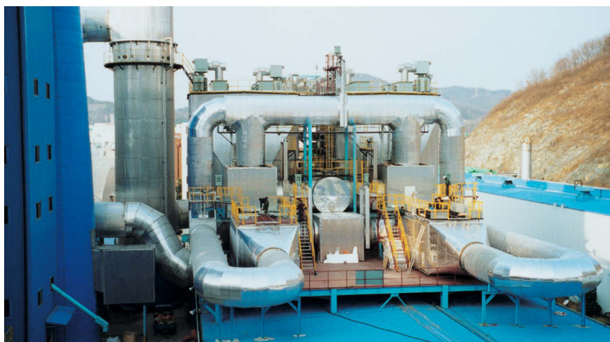
DeNO x catalytic system for glass smelter; 2 x 152,300 m 3 /h
