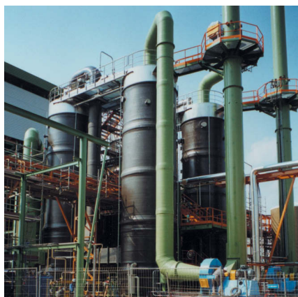
2 lines with a two-stage WESP each with special FRP casing and high degree stainless steel internals behind liquid waste incineration, quench and scrubber, volume each 37,000 Am 3 /h, efficiency > 99,5%
