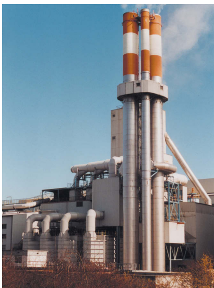
Horizontal electrostatic precipitator for curing oven and forming plenum waste gases each 100,000 Am 3 /h
