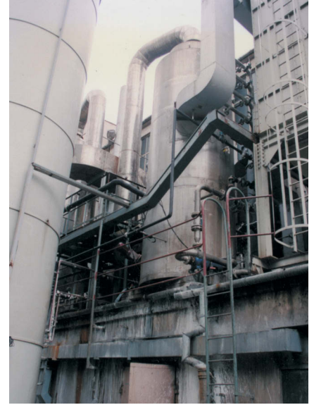
Flue gas desulphurization plant with spray tower, 25,000 m 3 /h, 200 °C
