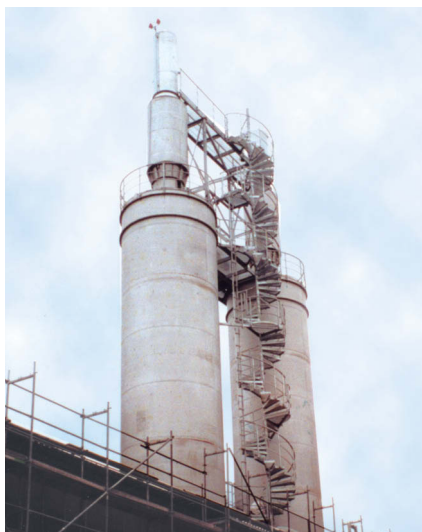
Two-stage WESP system behind forging press with integrated ultra-filtration for recyclable material
