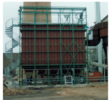
Bag filter with dry sorption in a thermal power plant with contaminated wood firing
