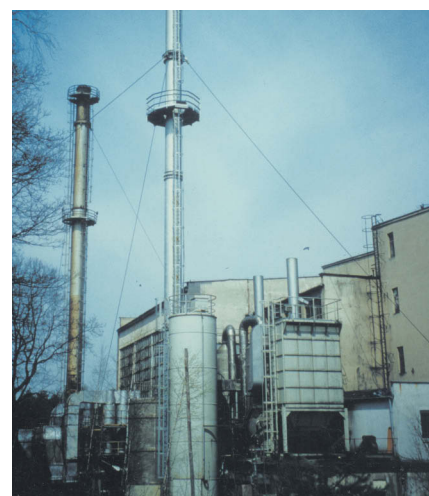
Mineral coal heating plant, combined installation system comprising exhaust gas heat recovery, flue dust collection and wet desulphurization
