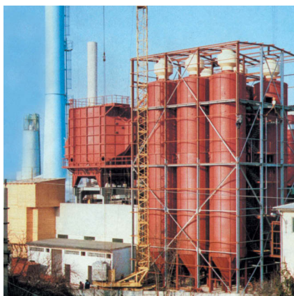
Wet electrostatic precipitator with biological water treatment system
