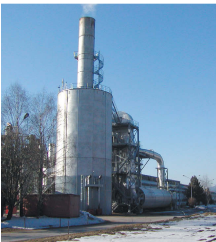
WESP behind a wood chip dryer, volume 300,000 m 3 /h, diameter 9,950 mm
