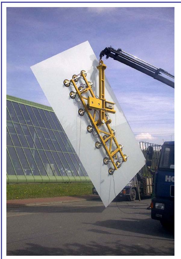
Architects and building owners are always making new demands on the glass processors. Large size sheets above the standard float glass measurement of 3,21 x 6,0 m are possible nowadays. And the glass processor cannot be surprised when even multiple laminated safety glass sheets having these measurements.
