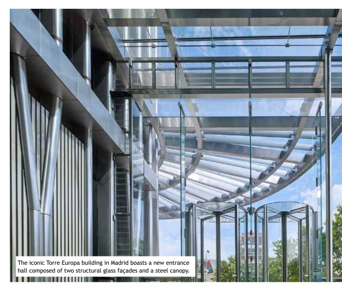
"The original design was done with PVB," Arbós elaborates, "and I was able to get good post-breakage performance from the PVB using the circular mounts, but when I did the same test using SentryGlas® the results were incredible. When the panel was broken, the PVB construction offered us about an hour of weight bearing before failure, whereas the SentryGlas® equipped panel simply refused to fail. Endesa was the beginning and we have kept using SentryGlas® ever since."
