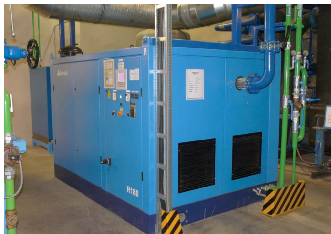
Saint-Gobain Oberland in Wirges uses two CompAir piston compressors to produce oil-free compressed air. This type of compressor is also widely used in breweries – an important customer sector for CompAir, Simmern.
