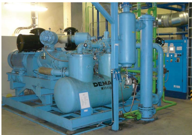
Four two-stage ROW 600 rotary vane compressors generate up to 15,000 m 3 /h of compressed air for the 6-bar network.
