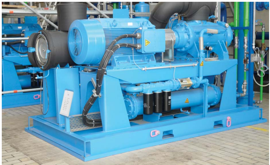
Rotary vane compressors from Gardner Denver Wittig generate compressed air for the 4-bar network.
