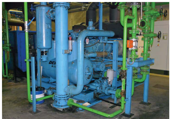
Vacuum air is generated by pump stations, which also operate under the rotary vane principle.
