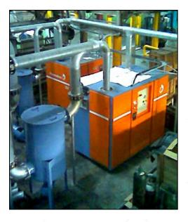
The collaboration with Malaya Glass started in 2004 when a new vacuum system for the Bottero IS machines was installed. Two pumps model UV8 and two model UV16 with all dedicated accessories operate continuously since then, at full customer satisfaction. The target of high-speed container glass manufacturing with a lowest rejection rate was achieved.
